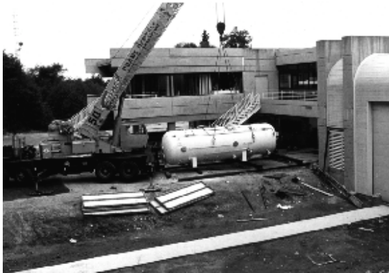
Figure 2: Installation of dive/altitude chamber.
