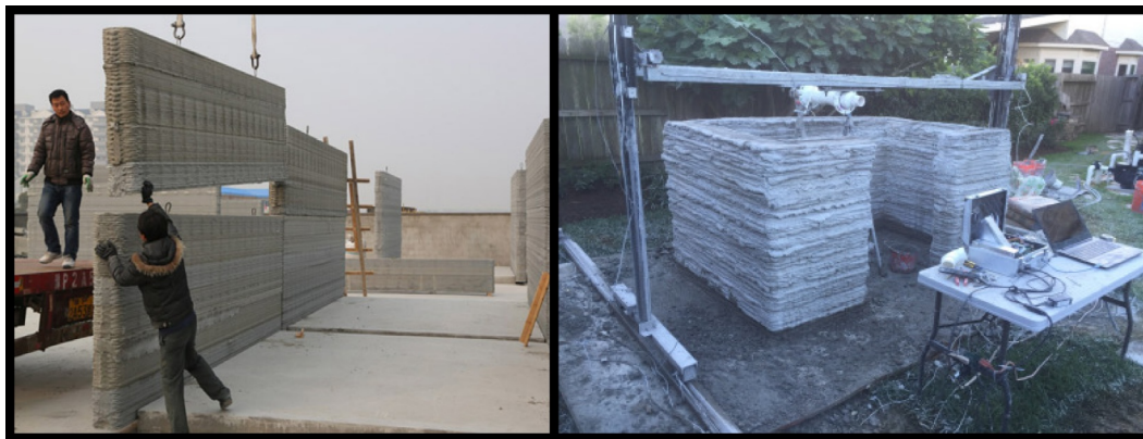
Figure 14: Example 3D printed concrete structure by industries worldwide [36,38]
